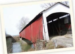
The Shieldstown Covered Bridge was the fourth and last covered bridge to be constructed in Jackson County. Built by J. J. Daniels at a cost of \$13,600, the two-span bridge was completed on November 17, 1876. The 355-foot-long bridge which spans the East Fork of the White River, has a multiple King Post design and utilizes the Burr Arch Truss system. The bridge carried traffic until the 1980's and is located approximately 1 mile north of U.S. Hwy. 50 W. on Co. Rd. 200 N.
